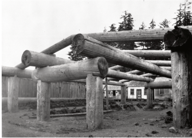
Figure 7.8 ▲ The framework of a large house with fluted beams in the Kwakiutl village of Mamalilikulla on Village Island, near Yalis (Alert Bay). Photographer Unknown. PN 1068, courtesy of the Royal BC Museum (1912).
